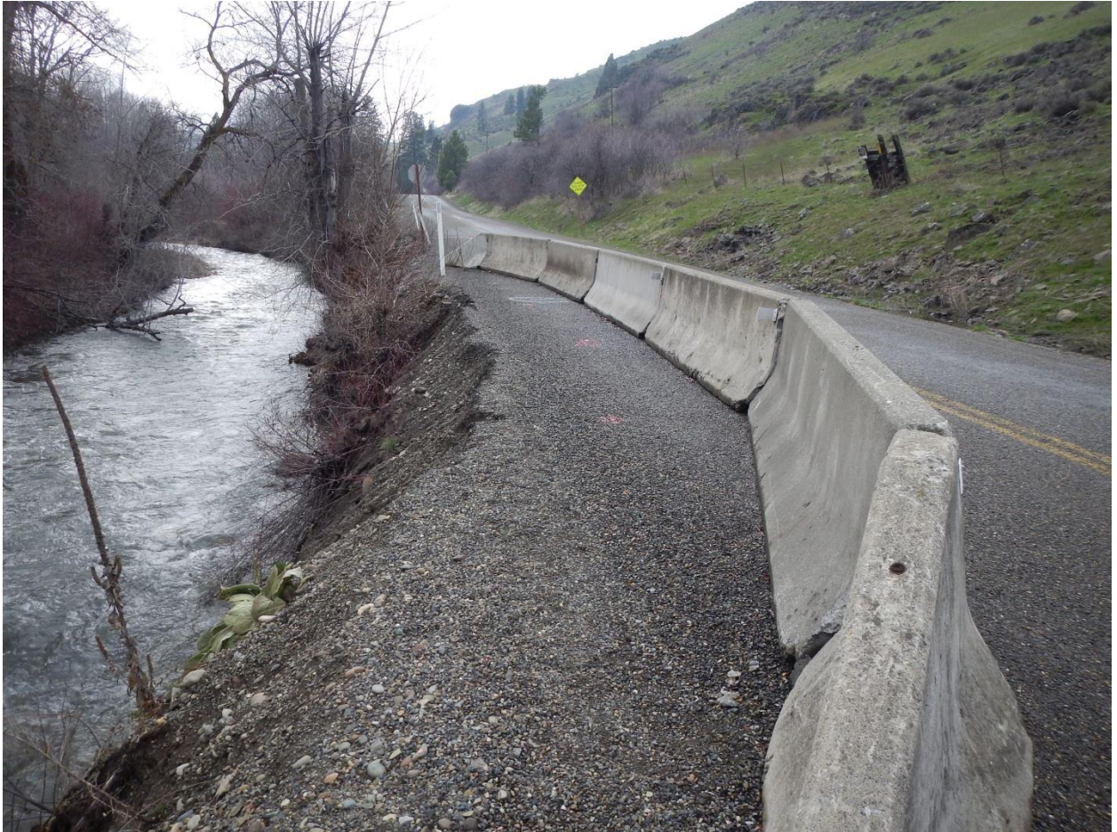
Southern Portion of the APE, View to the Northwest
