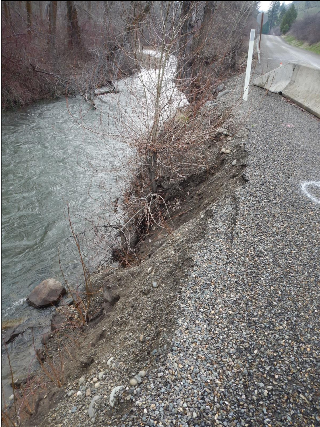
Overview of APE, View to the Southeast
